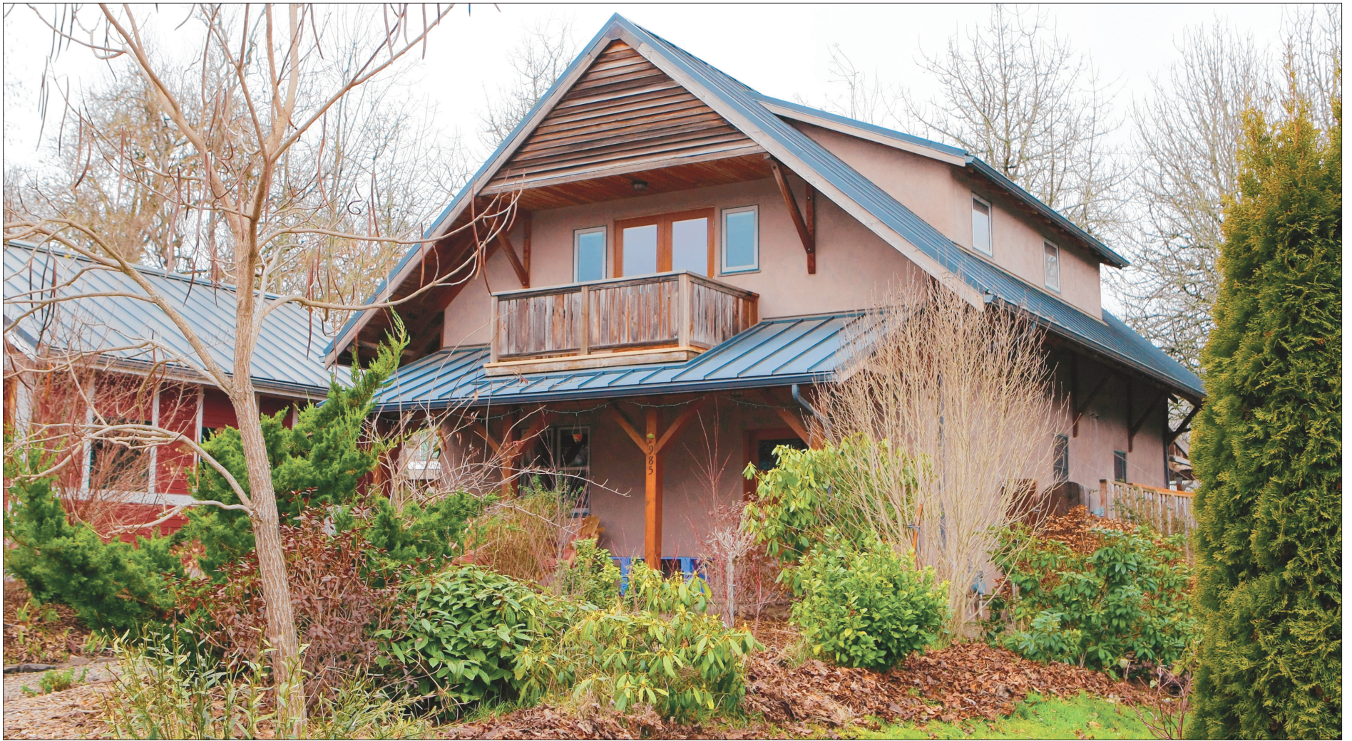
A hybrid of straw-bale construction and timber framing, this Eugene home has a long-lasting metal roof and deep overhangs to keep moisture away from the super-insulating straw inside its walls.
